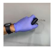
Open one pack of Sugru Moldable Glue. This is used to protect the epoxy from UV and environmental degradation. Roll the glue into a long enough cylinder so that it can be laid around the edge of the PinHold edge. Push the Sugru into the crevices and smooth out with your finger.
